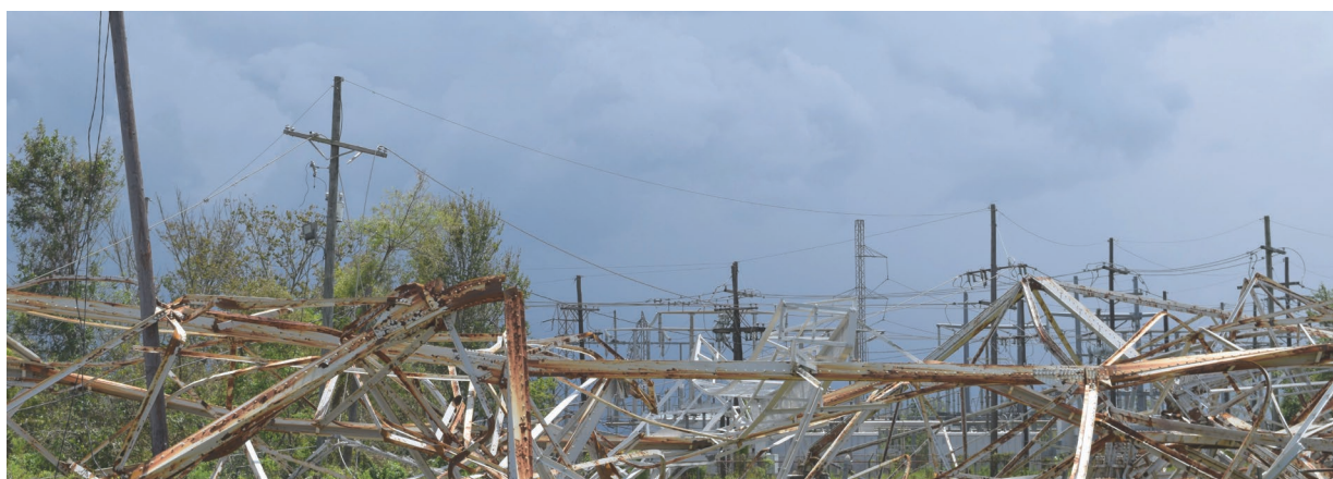
Figure 4. Collapsed transmission tower near Bridge City. 1
